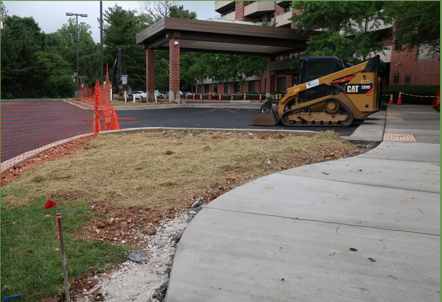
Front Entrance and Entryway Paving Near Completion
